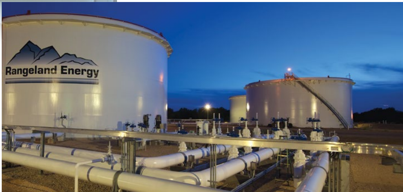
Night falls on Rangeland’s Geneva Terminal. The firm’s Geneva and Zurich terminals, located in Midland, Texas, provide valuable storage, terminaling services and connectivity to interstate pipelines that access the Cushing, Okla., trading hub; East Texas; and Gulf Coast markets.
